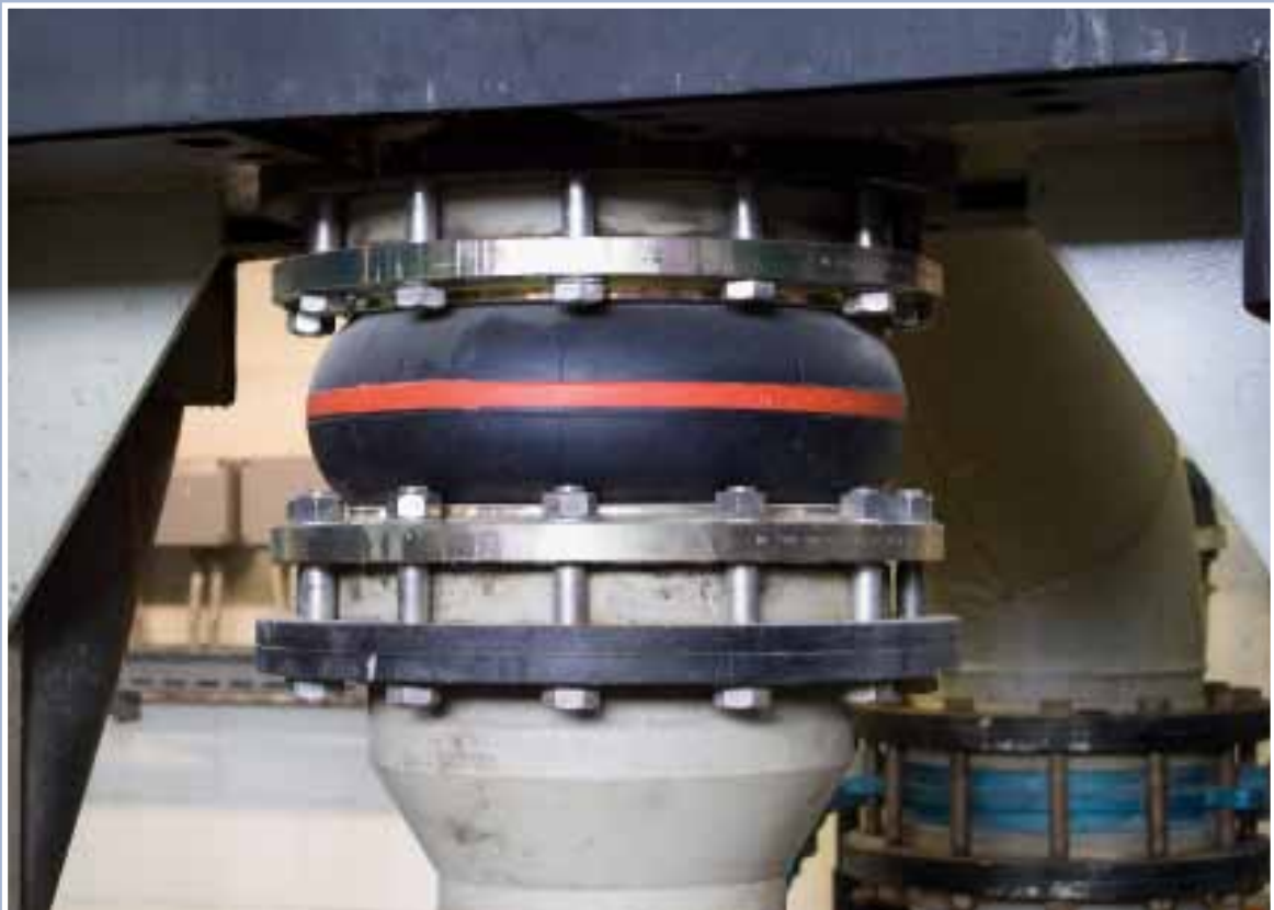
Universal expansion joint, type D110A in a GRP-pipe NB 250, 16 bar
