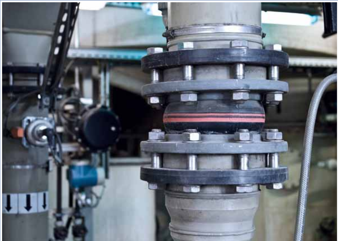
Universal expansion joint, type D110A in a GRP line NB 100, 16 bar
