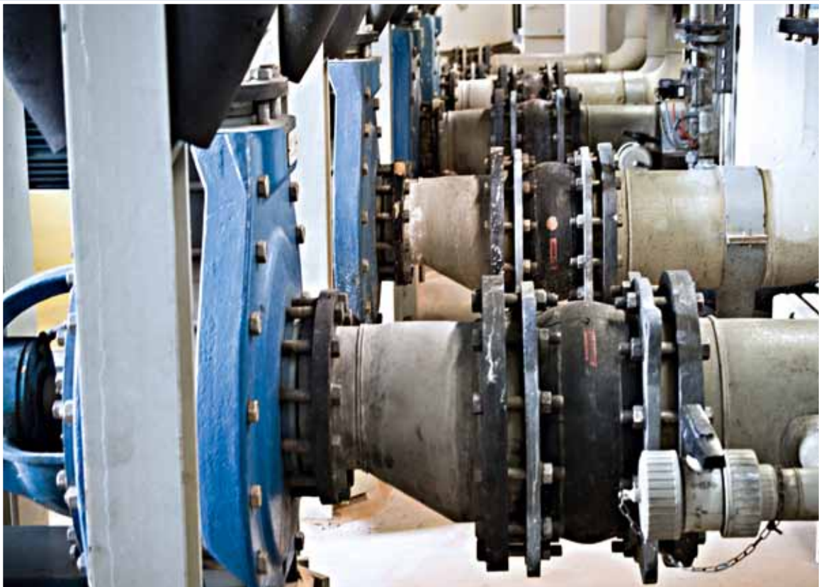
Universal expansion joint, type D110A on the pump's suction side NB 250, 10 bar
